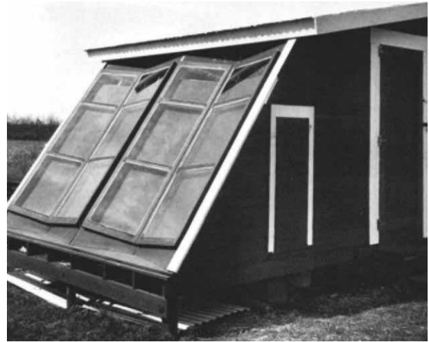
Solar panels on Johnson's kiln are tilted to catch early morning and late afternoon rays. Small door gives access to rear of solar collector, large door to stickered lumber.
